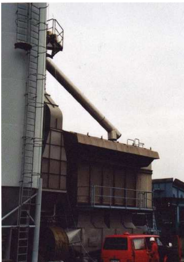
Figure 5 CO 2 Measurement at the plant
