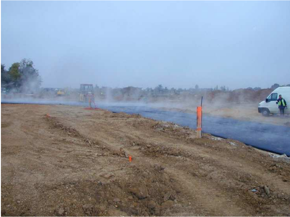
Figure 7 Construction of standard mix in France at 150 °C.
