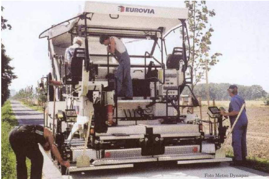
Figure 1 Construction site with AC 0/11 + aspha-min®
