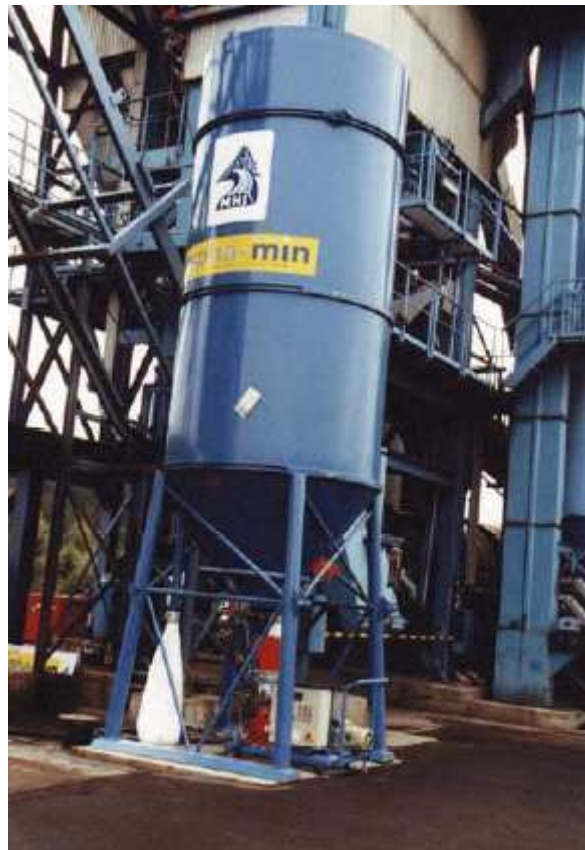
Figure 2 Adding the aspha-min®
